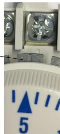
Replace the thermostat cover and tighten the securing screw on top and switch on the power to the control panel. Continue to monitor the operation of the pumping system to be assured that the pump is switching on and off at a point above the freezing point of water.
