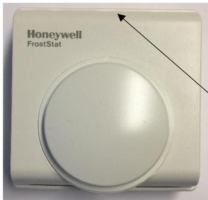
Accurate setting of the frost thermostat is difficult unless the air temperature is at the switch-on point, so it is factory set at 5°C. If the pump is switching on at too high a temperature, the thermostat can be adjusted.
